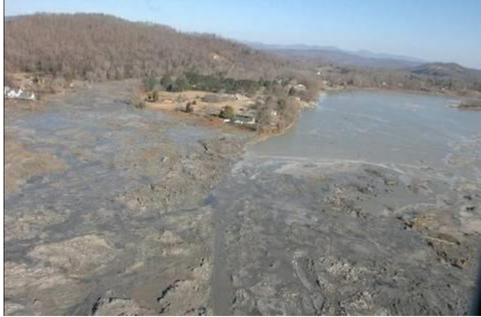
Figure 1.19: Ash sludge released from containment dikes in Kingston (EPA, 2009)
