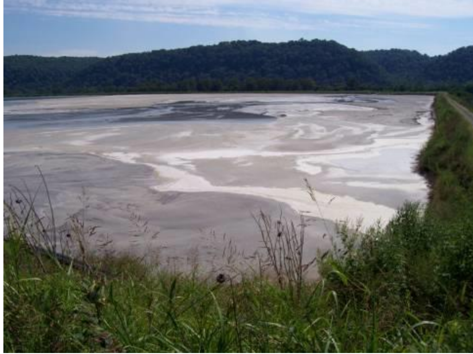
Figure 1.4: Wet disposal storage pond in Ohio Power Plant
