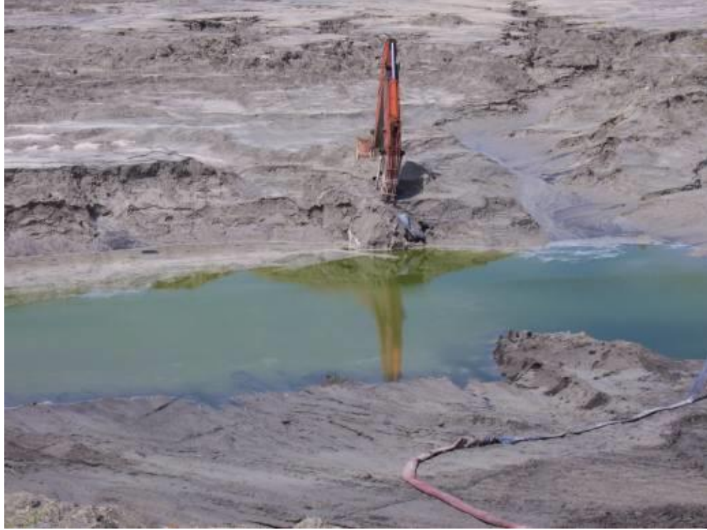
Figure 4.9: Storage pond failure at a power plant in Ohio
